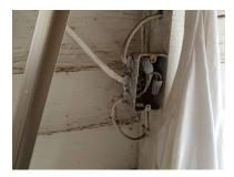
Branch wiring is loose. We recommend re-attaching the wiring to the joists / studs with proper staples / clips.
