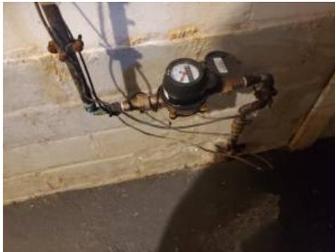
**DESCRIPTION:** Main water supply line is copper pipe.
