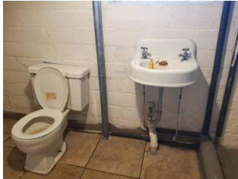
**FLOOR:** Flooring is covered / partially covered with ceramic tile. The condition of the sub-floor under the finished flooring could not be determined. Typically, when finished bathroom floors are replaced there is some water damage to the subfloor. We recommend budgeting for repairs to the sub-floor when estimating costs for replacing the flooring material.
